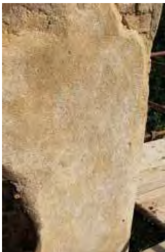
Figure 6: Plaster treated twice with CaLoSiL® E25.
