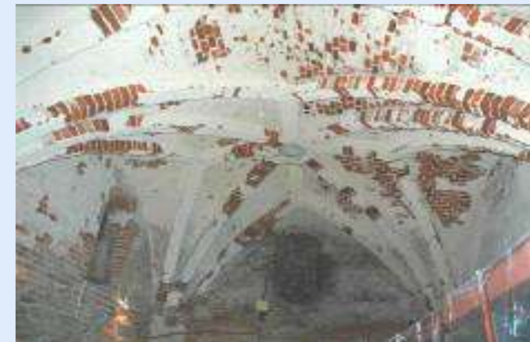
Malbork, (Poland); Consolidation of disintegrated medieval plasters; Realisation: Restaurow (Poland)
